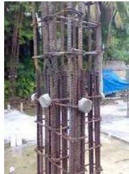
**Gambar 3.11** Kolom beton
